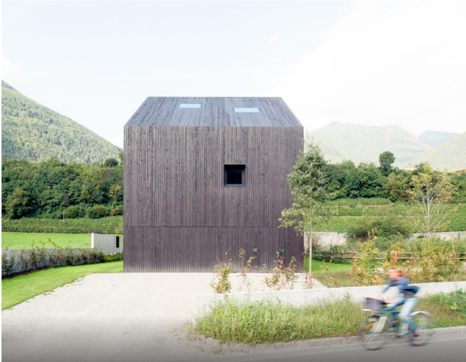
REFERENCE: EXTERIOR WOOD CLADDING DETAIL SHOWING CONTINUOUS INSULATION + WATER-PROOFING LAYER UNDER CLADDING
